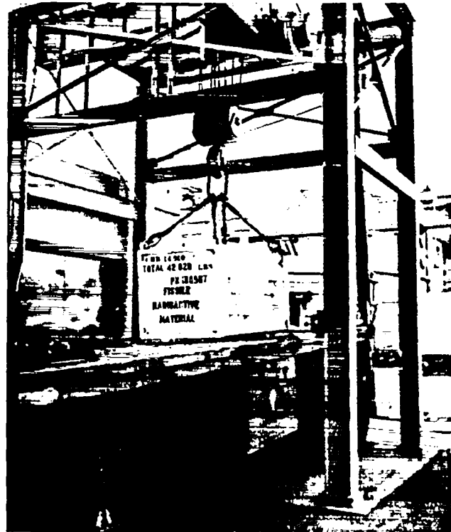
Fig. 401-2. 25-Ton Hoist at DP West Hot Cells.
